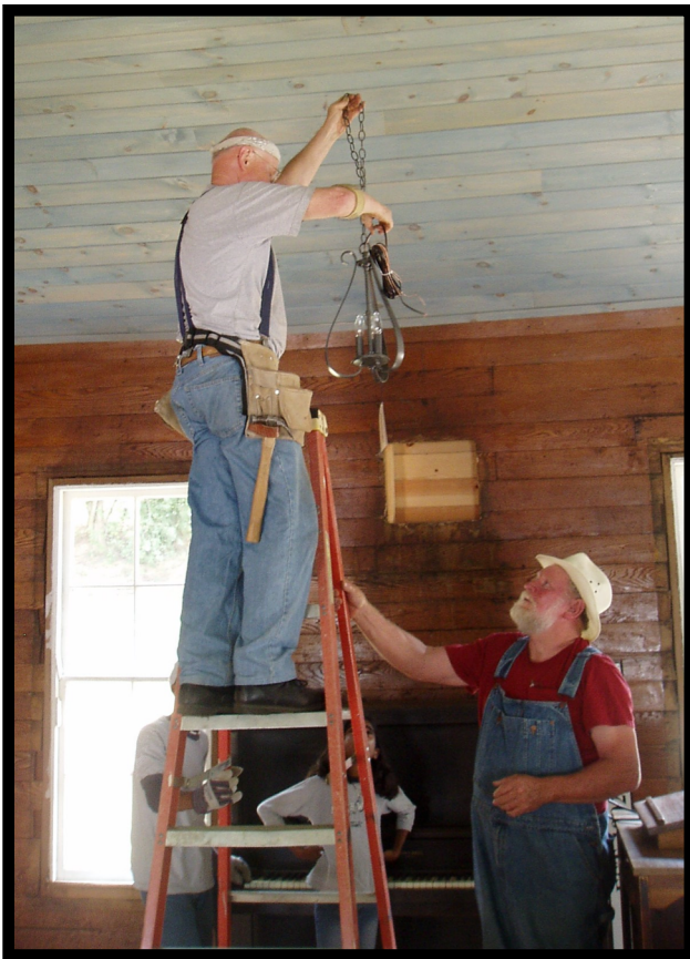
David Reese helping Bob install new light fixtures.
