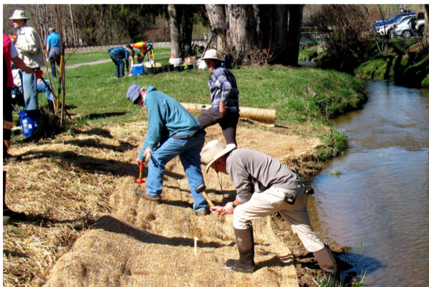
Participants at the Streambank Enhancement workshop helped scatter grass seed and pound live stakes into the streambank. The grass will emerge through the mulch during April, and the live stakes should be growing and leafing out by this summer.
