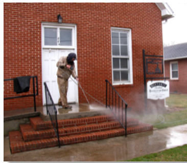
Power washing the church entrance
