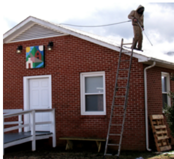
Removing the roof moss
