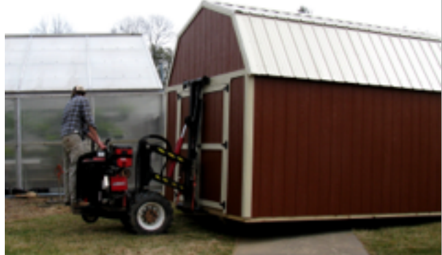
Because there are "rollers" beneath the storage unit, it is easy to pull it across the grass.
