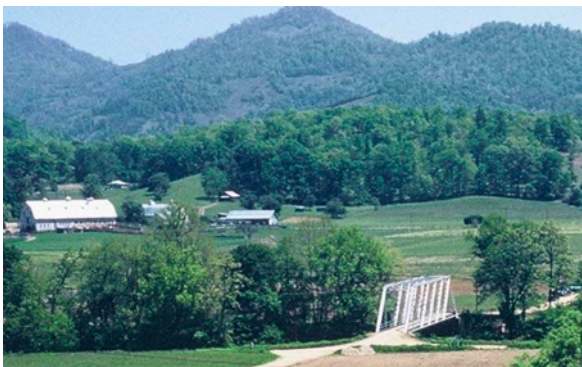
Wells Road bridge
